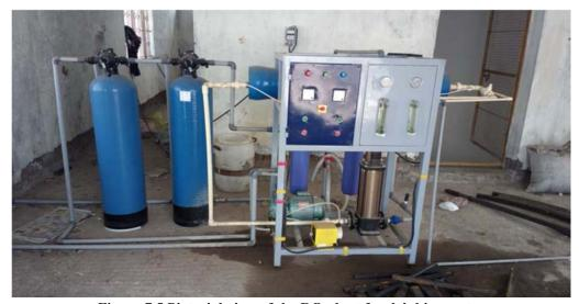
Figure 7.5 Pictorial view of the RO plant for drinking water
